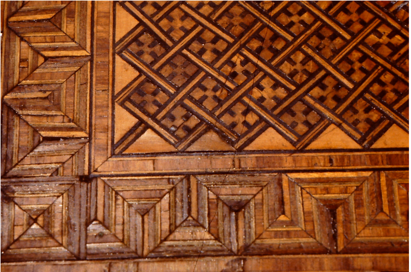
Figure 7: Detail of a marquetry surface after rehydration, showing expansion of original mastic, and slight deformation of wood elements, ready for application of modified animal glue.
